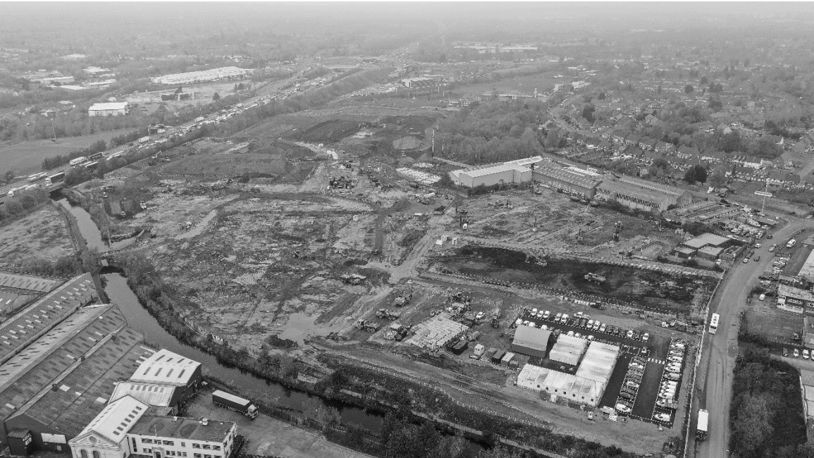
Figure 1 – Aerial photo of work on site
