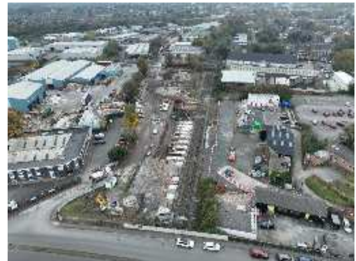
Willenhall aerial view of progress
