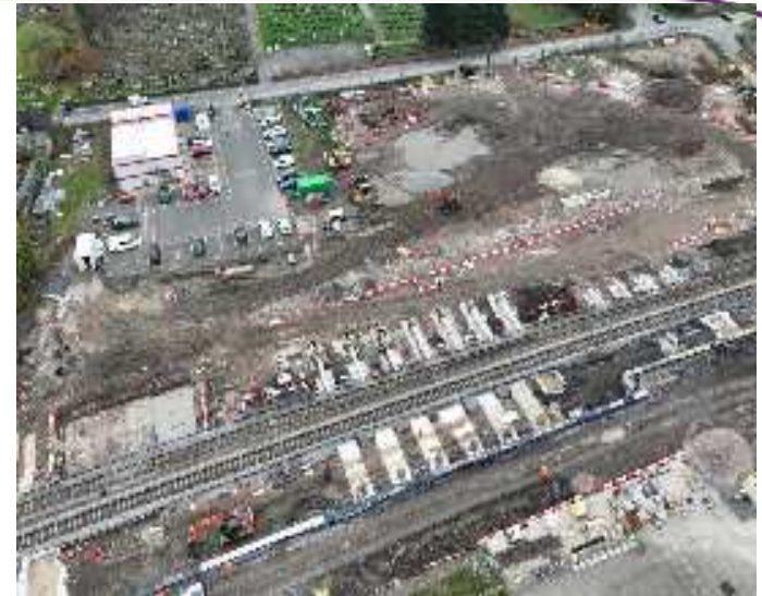
Darlaston aerial view of progress
