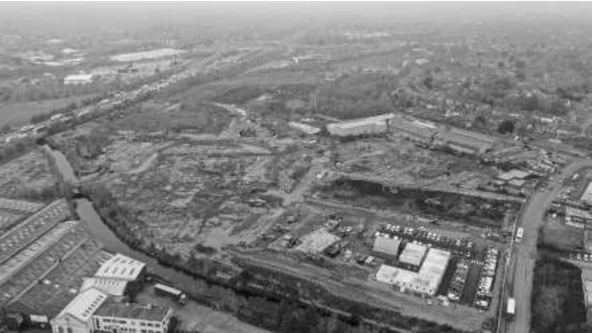
Figure 1 – Aerial photo of work on site
