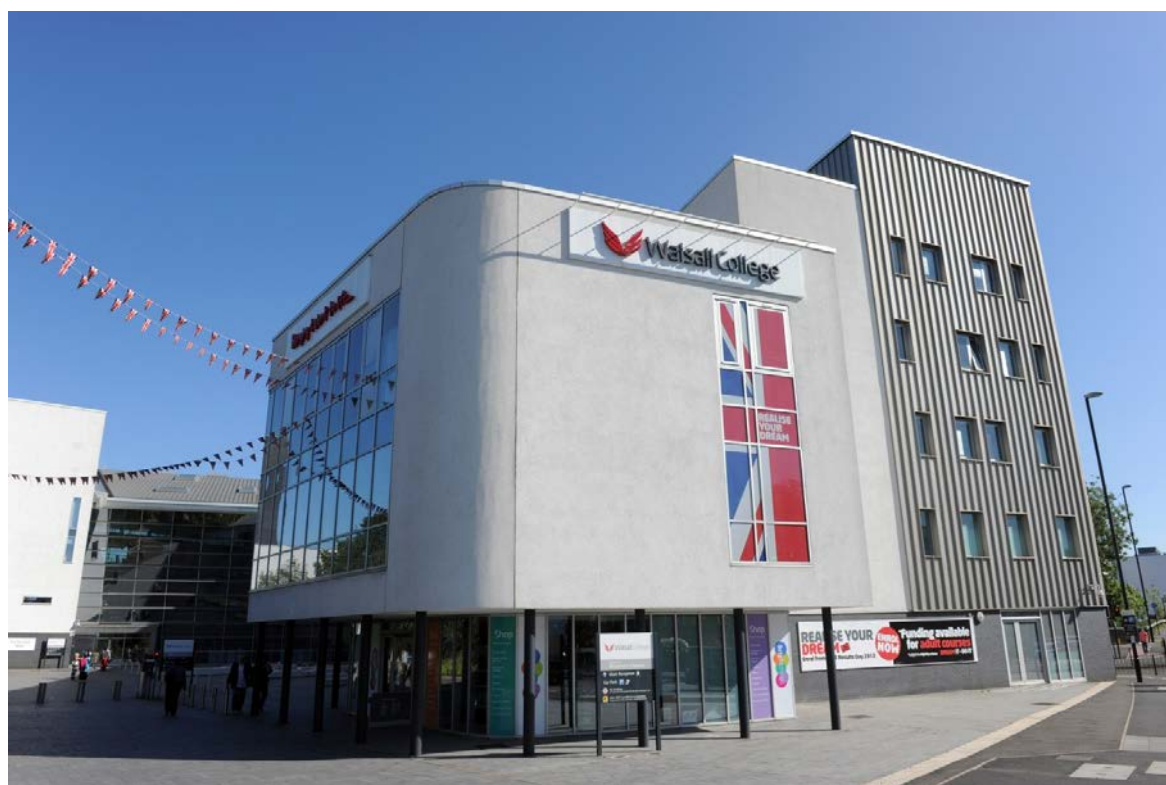
Figure 6.1 Walsall College, Littleton Street West
