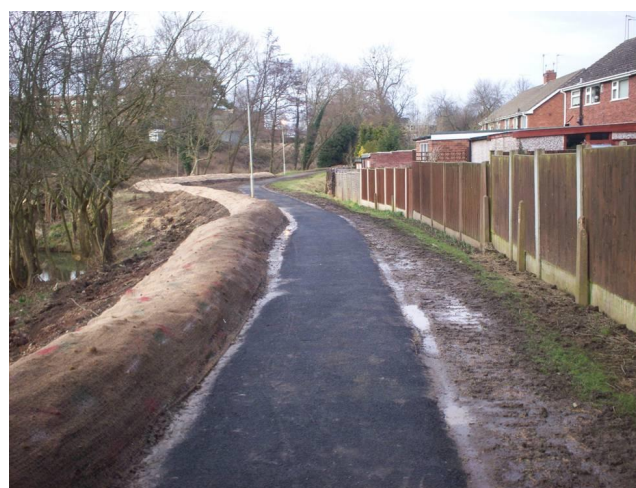
Figure 3 - Defence bund and wall installed adjacent to River Stour at Grange Crescent, Halesowen in 2012, in partnership with the Environment Agency
